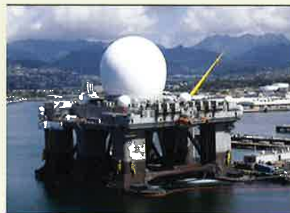
The Sea-Based X-Band Radar (SBX-1) is a floating, self-propelled, mobile active electronically scanned array early-warning radar station designed to operate in high winds and heavy seas. It was developed as part of the Missile Defense Agency's Ballistic Missile Defense System. The radar is mounted on a fifth generation CS-50 twin-hulled semi-submersible oil platform. Conversion of the vessel was carried out at the AmFELS yard in Brownsville, Texas; the radar mount was built and mounted on the vessel at the Kiewit yard in Ingleside, Texas. It is nominally based at Adak Island in Alaska (though, as of April 2015 has never put into port at Adak). It has spent significant time at Pearl Harbor in test status.
